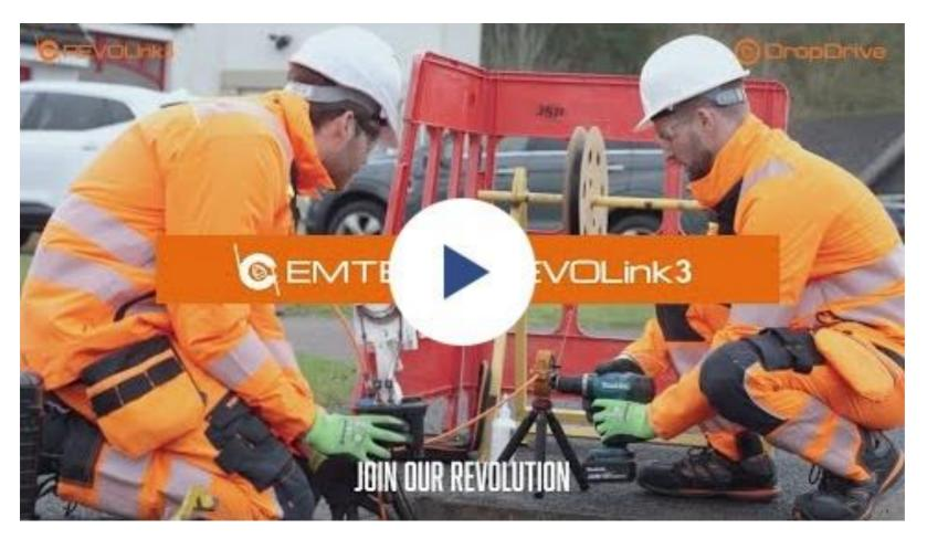
Introducing another innovation by Emtelle, the Ultimate Drop Cable Solution, a revolutionary pre-connectorised cable and drill-assisted pushing machine, designed for the ultimate performance. In the high-demand world of FTTh installations, challenges such as soaring splicing costs, the demand for skilled labour, limited warehouse space, and a scarcity of fibre installers have propelled the guest for a transformative solution.
